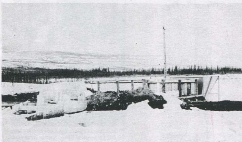
This recent arrival to our view of the McQueston Valley is a feeder for the Lime that is being added to the Settling Pond to provide better control of Mill effluent.
