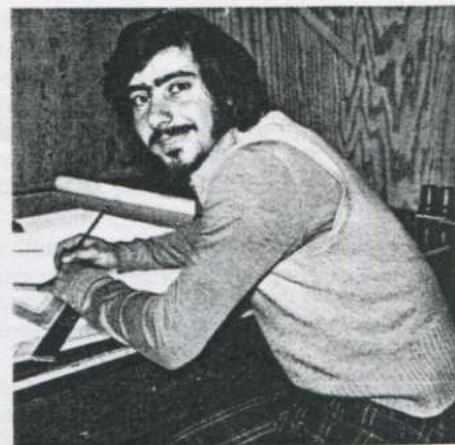
Draftsman Peter Alfano. After Peter receives the assay reports on overburden drilling, he plots the drill holes on a map. Then he makes a section of each individual hole, showing the amount of lead and silver for every five feet drilled. Geologists Jim Ellerington and Terry Levicki examine each cross-section to decide whether or not it is worthwhile doing more drilling in that area. (Peter says his biggest headache is his sore back.)
