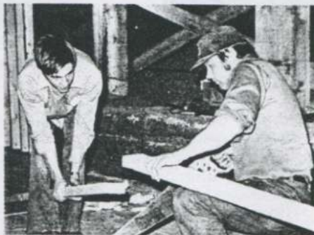
Norman Case and Ralph Mease are busy sawing boards for the floors in the Hockey Club's dressing rooms underneath the Rec Hall. The Lions Club started the project two years ago. However, only a pit was dug. This year the Hockey Club got the ball rolling, and many people are helping. After completion, there will be two rooms, each thirteen feet wide, sixteen feet long, and six-and-a-half feet high. One room will be used to store Hockey Club equipment. The other will be open for skaters to change and warm up.
