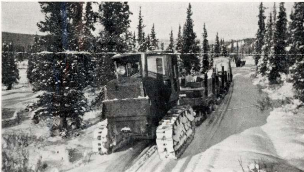
Treadwell-Yukon Company, Limited, Tractor hauling ore from the mine to Mayo Landing.
