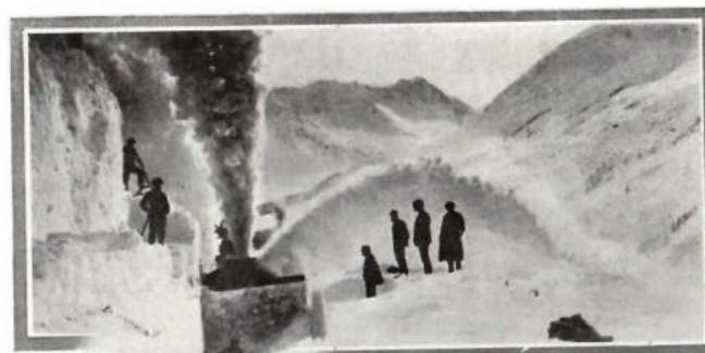
High In The Mountains During Winter Rotary Snow Plow at work on W. P. & Y. R.
